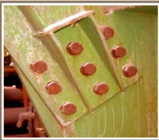
Badly Corroded
